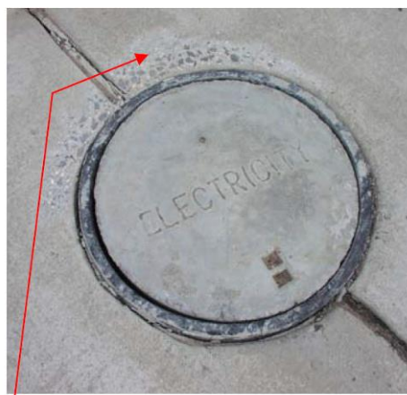
Figure 50 - Acceptable - Grinding of Footpath
