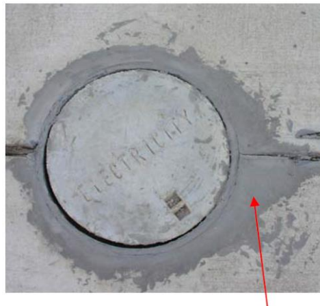
Figure 49 - Non-Compliance – Use of Filler
